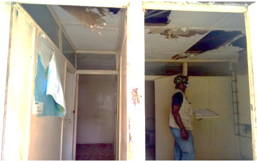
Before: asbestos in roof
