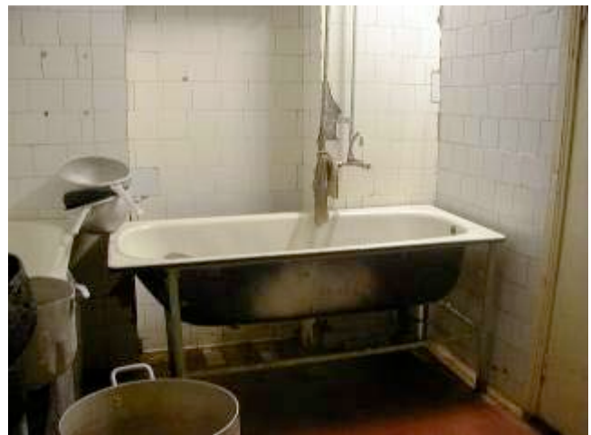
The only facility for washing kitchen utensils and hands in a hospital kitchen in Eastern Europe.
