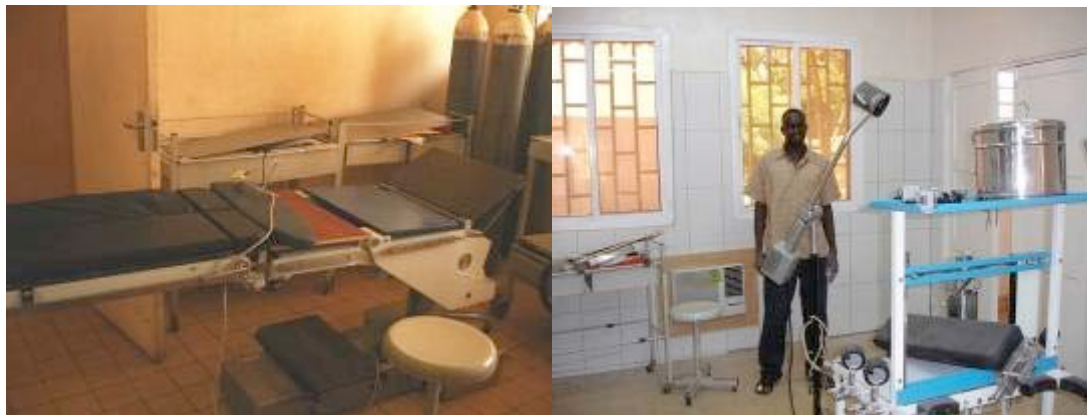
An operating theatre in rural Gambia before and after renovation
