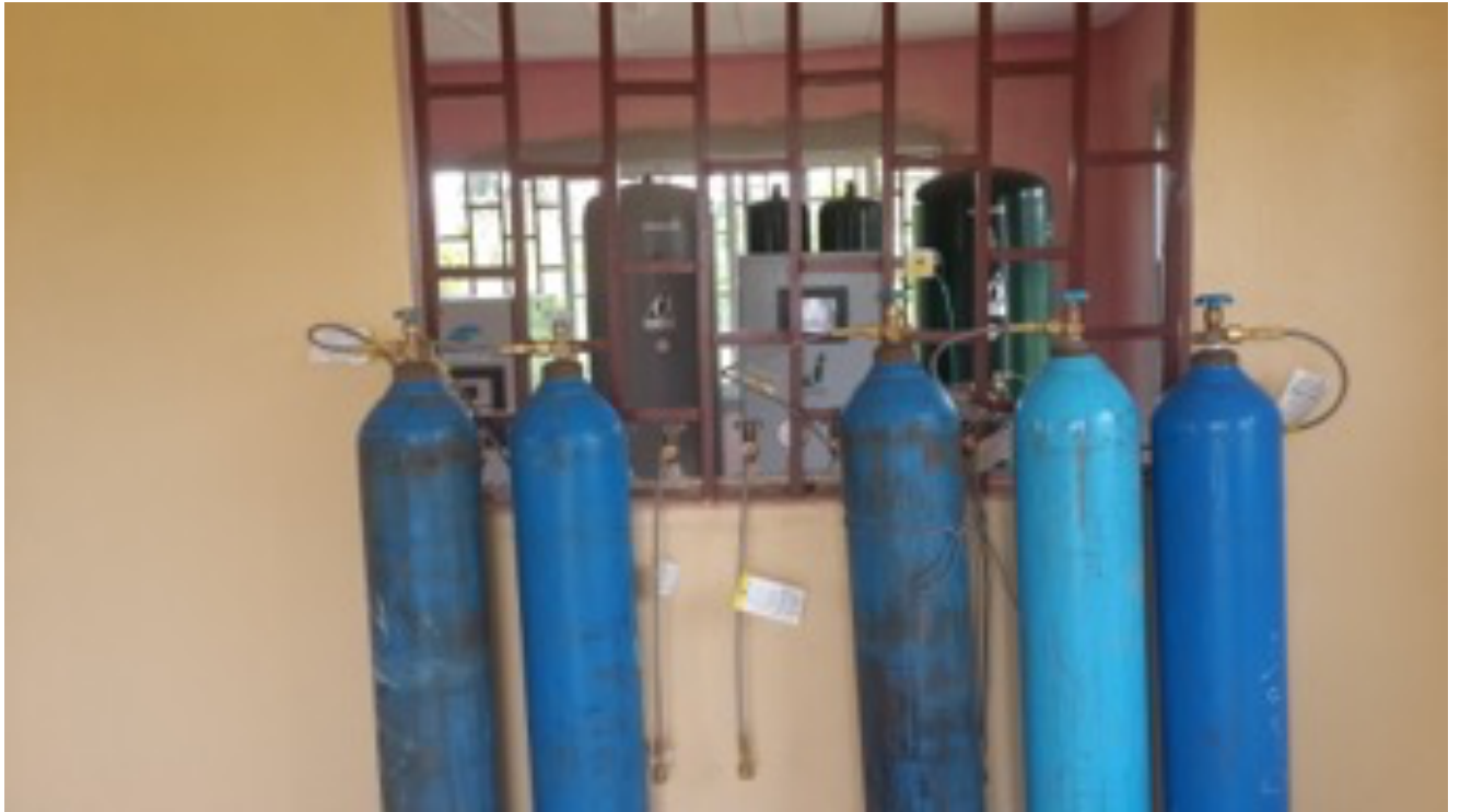
ABOVE: Because of the unreliability of electrically powered oxygen supply systems (oxygen concentrators), during the Ebola outbreak, MCAI provided an oxygen generator system based at Phebe Hospital that produces large cylinders full of medical grade oxygen for 4 nearby hospitals, including CB Dunbar Hospital
