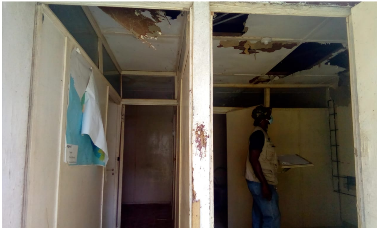
UNDER CEILING TILES BETWEEN ISOLATION WARD AND MALNUTRITION UNIT IS ASBESTOS
